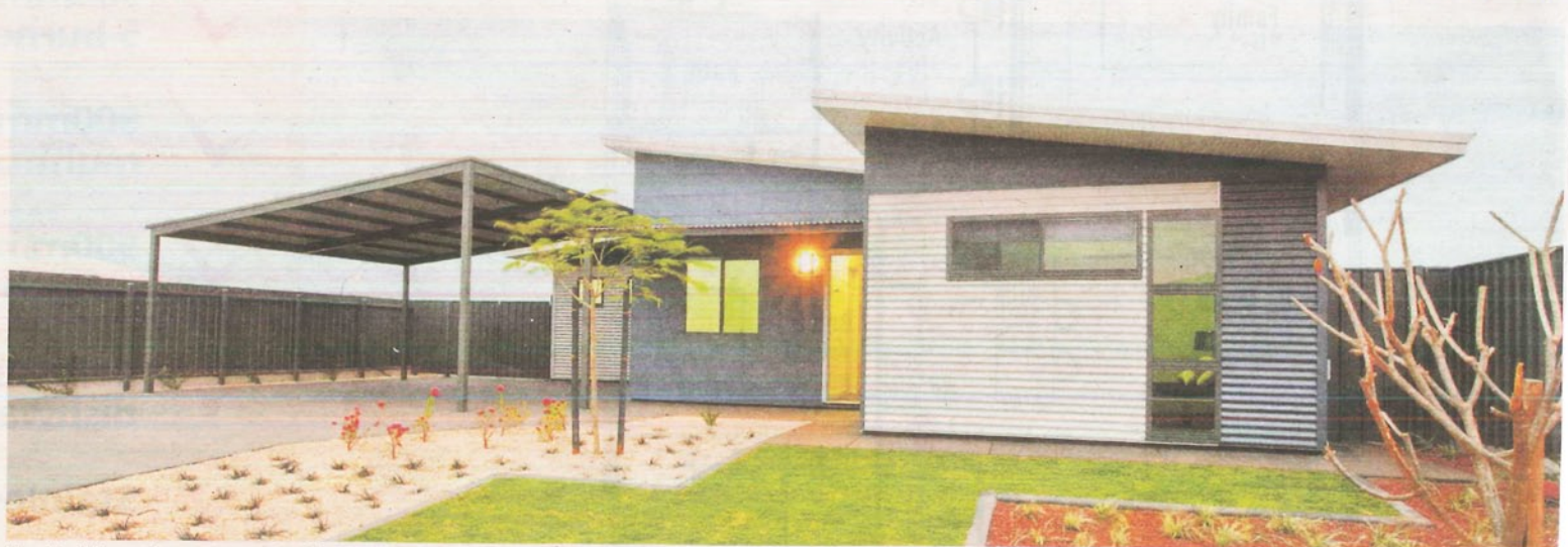
The Residence has a concrete floor with engineered steel-framed walls and roof.
